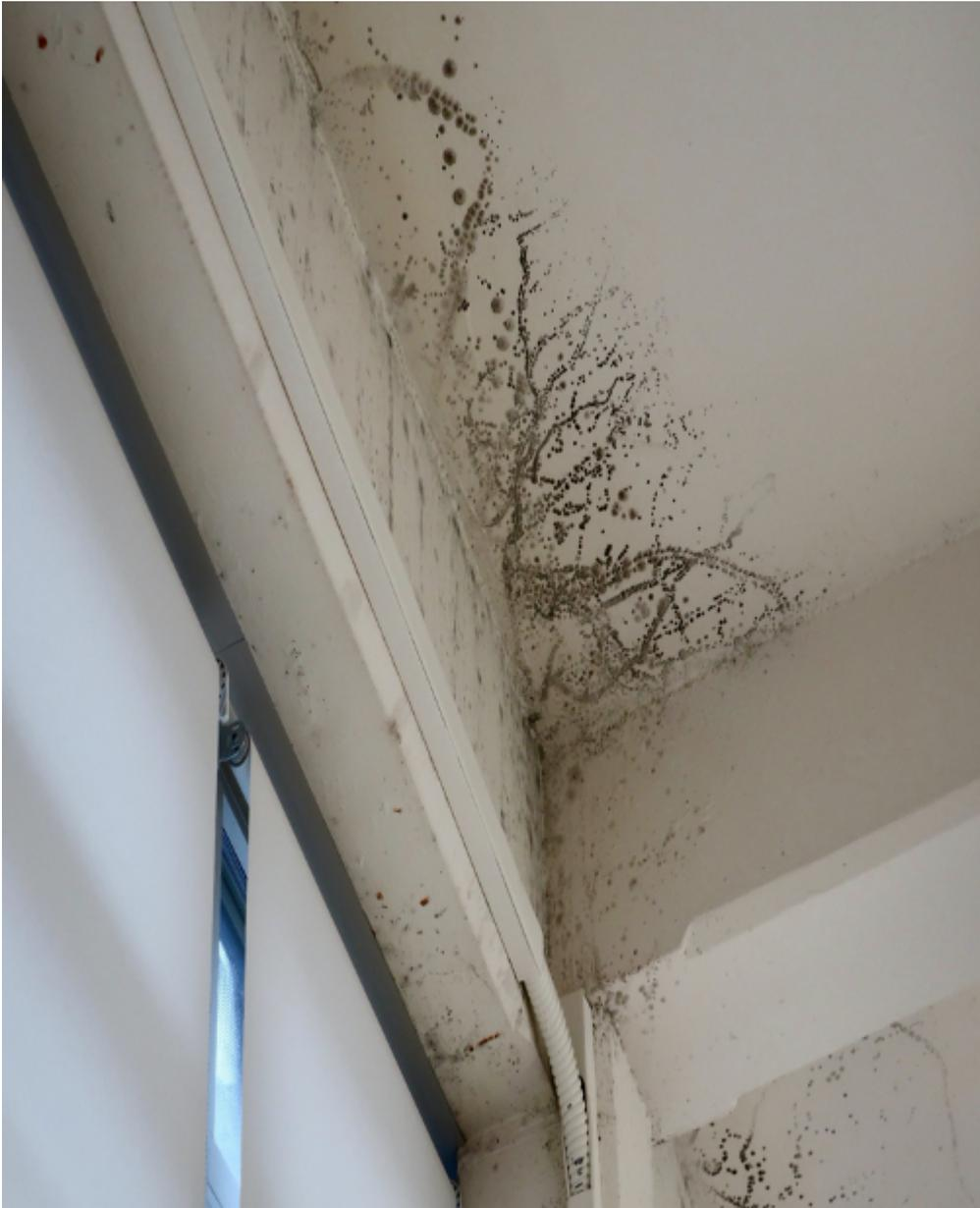
**Photo 14 - ES Library – Mold growth on ceiling associated with ongoing and uncontrolled steam leak**
