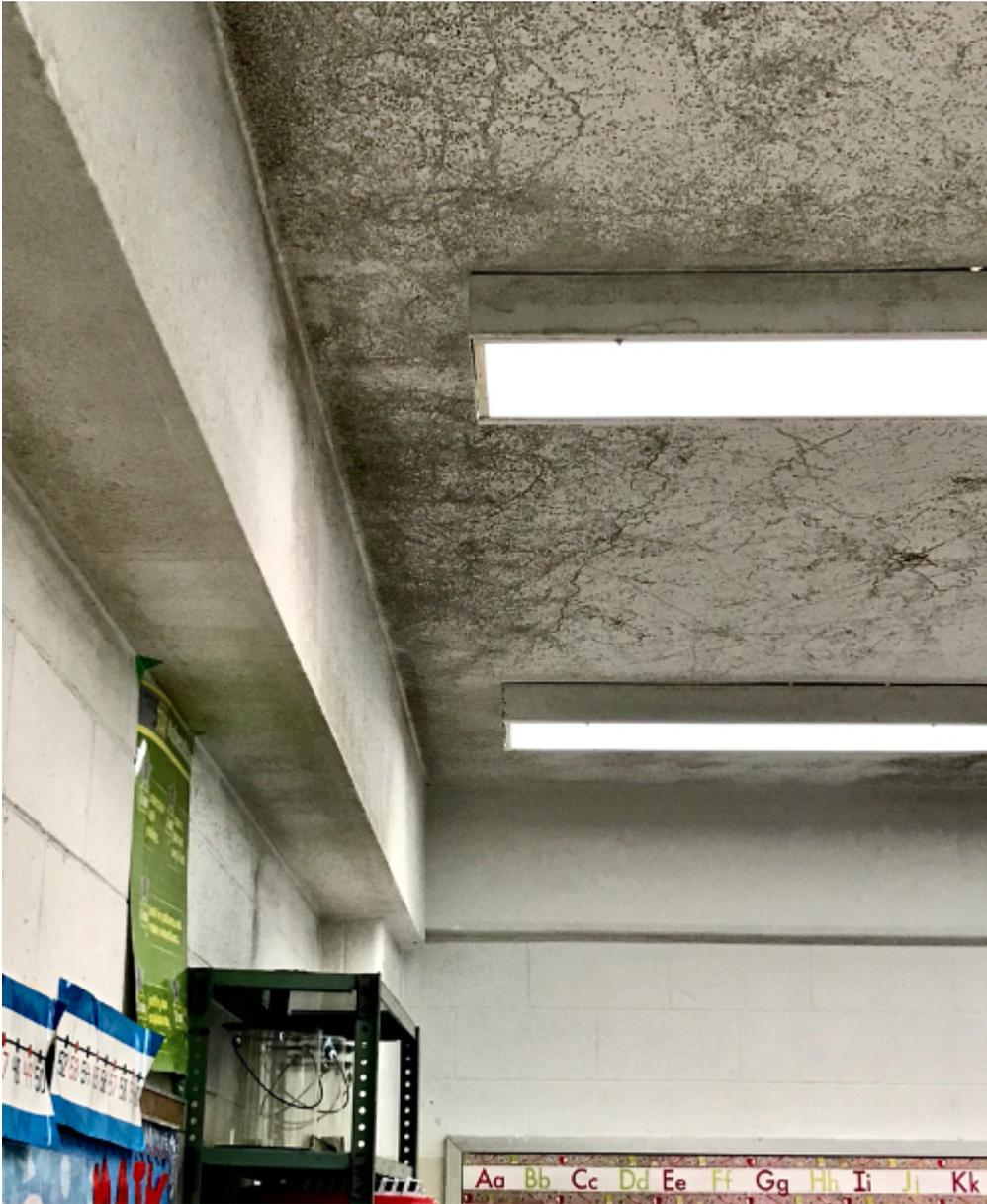
**Photo 6** – Close up (of photo above) of Mold growth on ceiling
