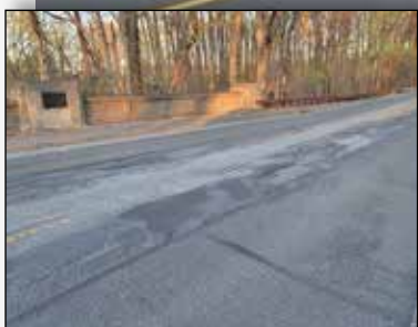
Rhawn Street before paving
